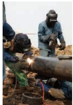
Pipeline Construction/ Maintenance
